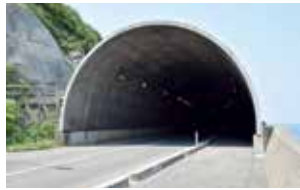
Tunnels and concrete pipes
