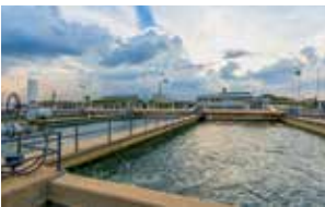
Collecting and retaining basins
