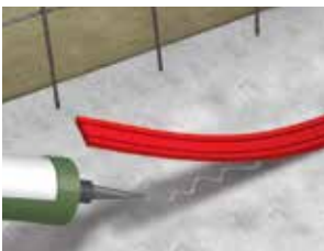
1. Bonding using a mounting adhesive
